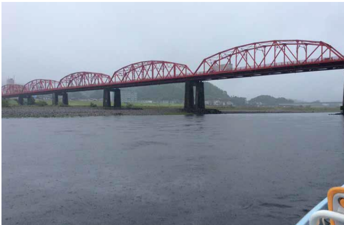
Akatetsu Bridge and rainfall viewed from the left bank to the right bank
